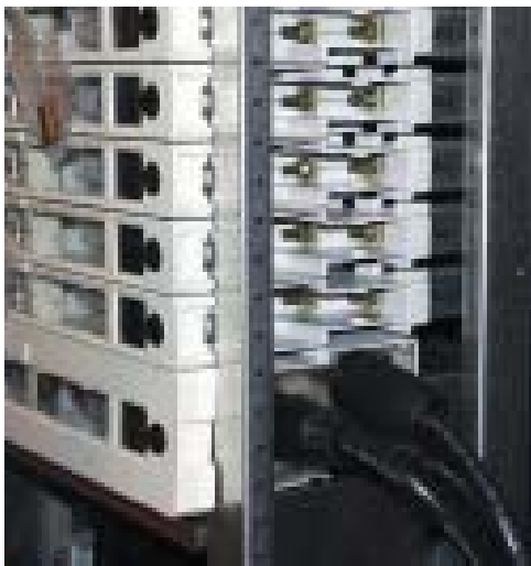
Slimline Switchfuse with outgoing cables
