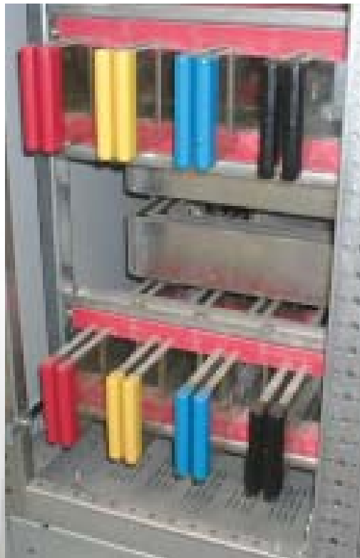
2 Tier main Busbars 6300A
