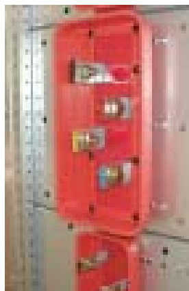
Outgoing terminals with boot retainer
