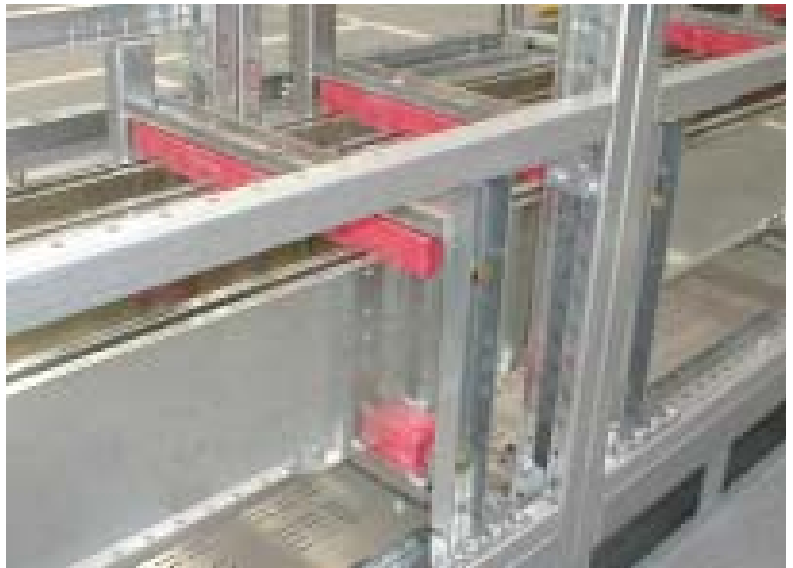
4000A main Busbars
