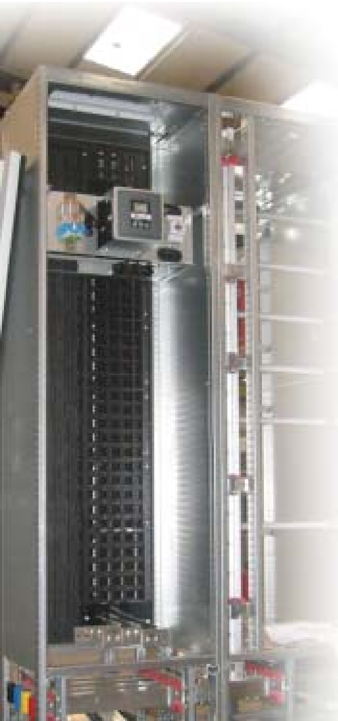
Multi-functional wall connected to main Busbars
