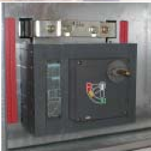
MCCB in cassette mounted in switchboard
