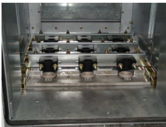
3 cables per phase 800 mm wide unit
