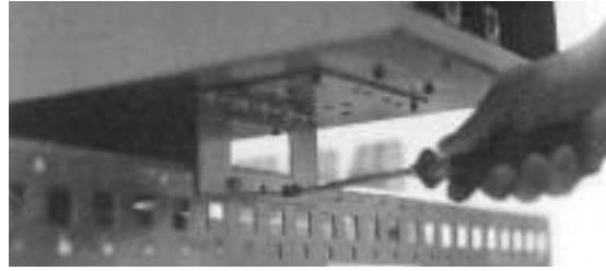
The fusible switch module has a self-aligning bracket screwed to the interior mounting rails.
