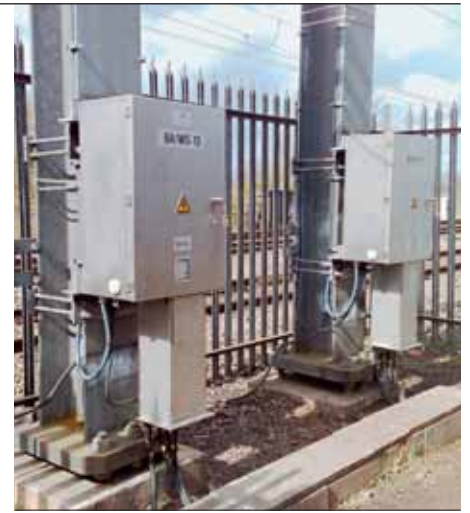
1b New electronic controller at ground level
