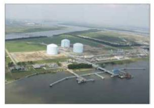
more cooling stages. Cooling work consumes 6-10% of the energy to be transported. Special insulated tank LNG carriers are required for transportation, and at the receiving end, a regasification terminal heats the LNG to vaporization for pipeline distribution. *Photo: Cove Point LNG Regas terminal*
