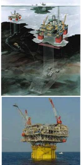
the bottom by a series of cables and lines. The large cylinder serves to stabilize the platform in the water, and allows for movement to absorb the force of potential hurricanes. SPARs can be quite large and are used for water depths from 300 up to 3,000 meters. SPAR is not an acronym, and is named for its resemblance to a ship's spar. SPARs can support dry completion wells, but are more often used with subsea wells.
