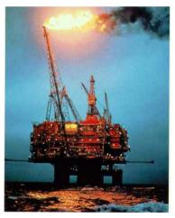
Stronger environmental focus has eliminated continuous flaring and the pilot in many areas. Vapors and flare gas are normally recovered, and only in exceptional situations does flaring occur. To avoid the pilot flame, an ignition system is used to ensure safe ignition, even when large volumes are discharged. One patented solution is a "ballistic ignition" system which fires burning pellets into the flare gas flow.
