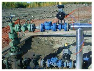
and temperature of the formation, and installing the proper equipment to ensure an efficient flow of natural gas from the well. The well flow is controlled with a choke.
