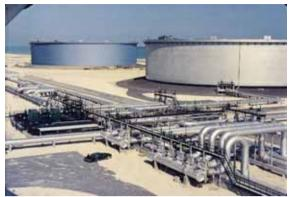
shuttle tanker to offload about once a week. A larger production complex generally has an associated tank farm terminal allowing the storage of different grades of crude to take up changes in demand, delays in transport, etc.
