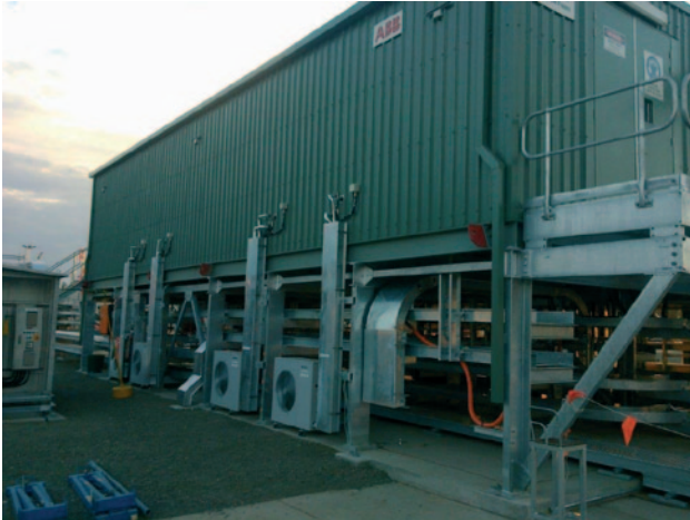
1. LNG Plant E-House Installation 3 Industrial Plant E-House Installation
