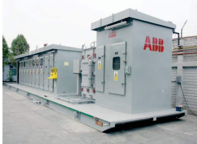
2. Power Generation Plant E-House Installation 4. Above Ground Mining Skid
