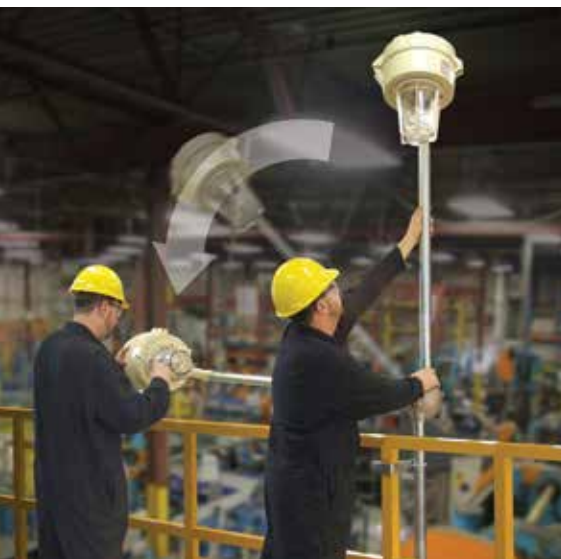
— 01 The quick pole assembly blocks at a 90° angle.
