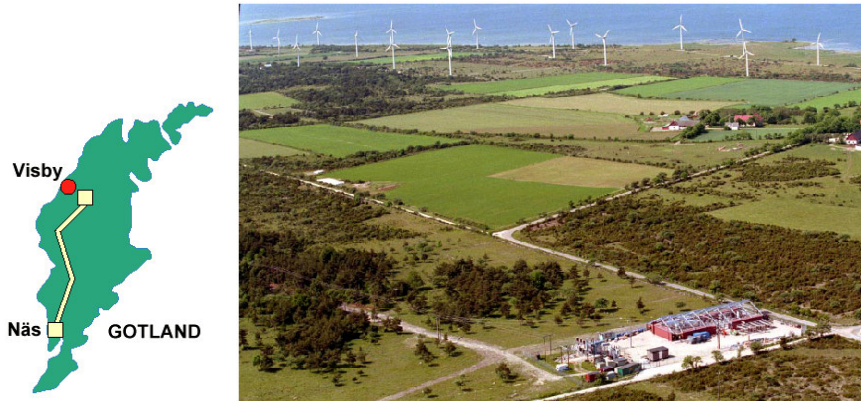
Figure 7. The first commercial HVDC Light cable system connecting a wind park on Gotland.
