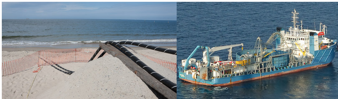
Figure 9. The photos above views the landfall of North Sea and the two 150 kV HVDC Light Cables, 1600mm 2 copper conductor, for the BorWin 1 project.
