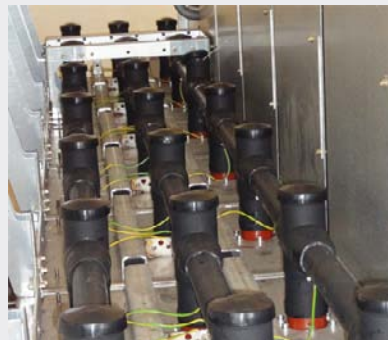
Busbar compartment with support for voltage transformers
