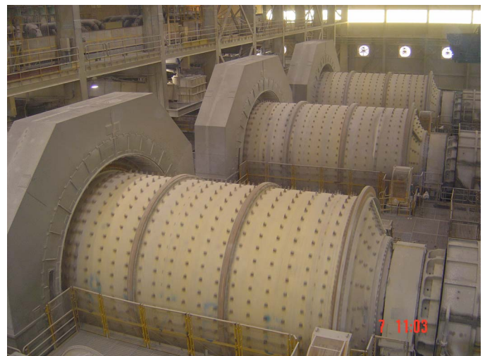
Figure 1. Picture of the Ball Mills at the Laguna Seca Concentrator
