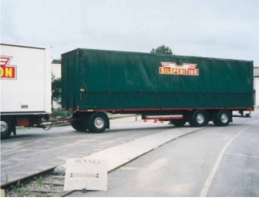
PFBC ash used as base material and as a sealing layer on the site of ABB Carbon in Finspong, Sweden
