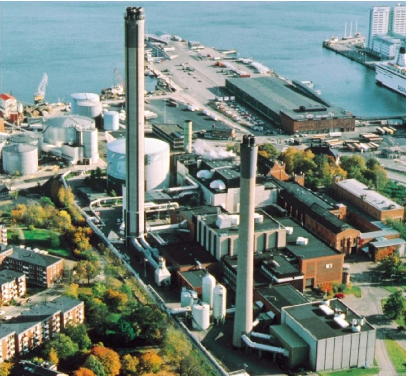
Värtan PFBC combined cycle power plant, Stockholm, with an electrical rating of 135 MW and a thermal rating of 224 MW
