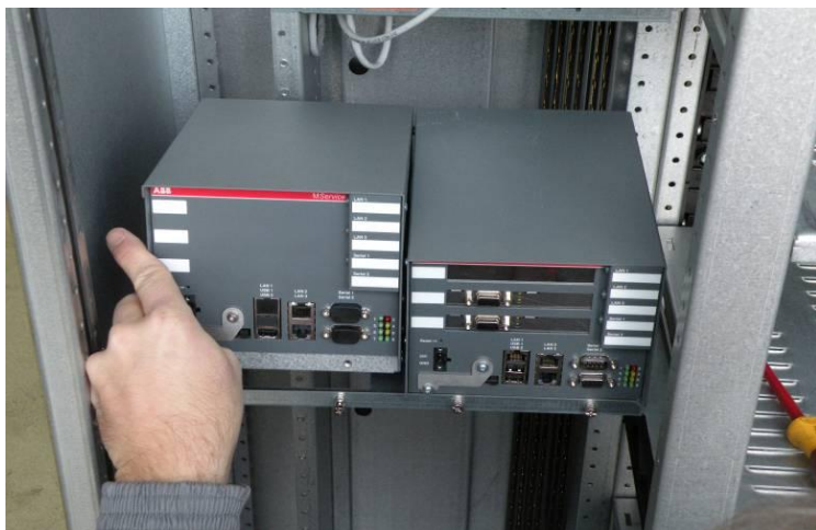
Fig. 3: Example of MService placement in MNS iS switchboard
