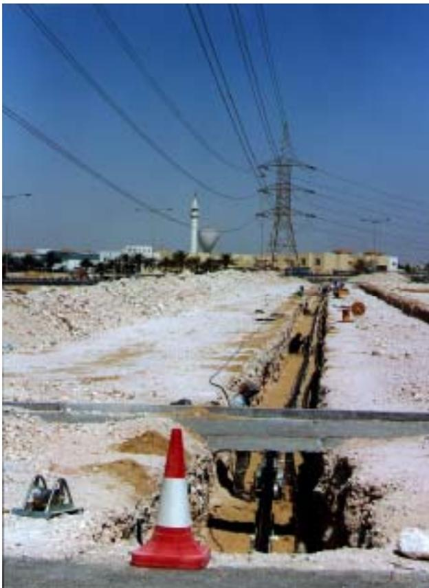
*Figure 7: Example of cable laying in a corridor already used by OH-lines. AC PEX-cable in Qatar.*
