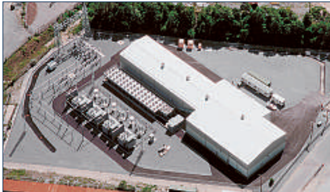
4 Shoreham is one of two converter stations of the Cross Sound Cable Interconnector, between Long Island and Connecticut.
