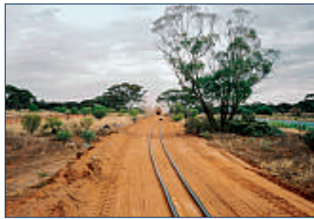
Laying cable for the Murraylink HVDC Light project, Australia, the longest underground power transmission cable in the world.
