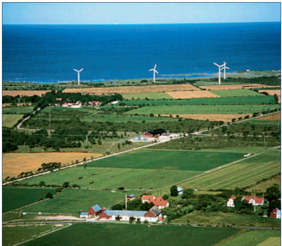
1 Näs Head HVDC Light station with the converter building in the middle of the picture.
