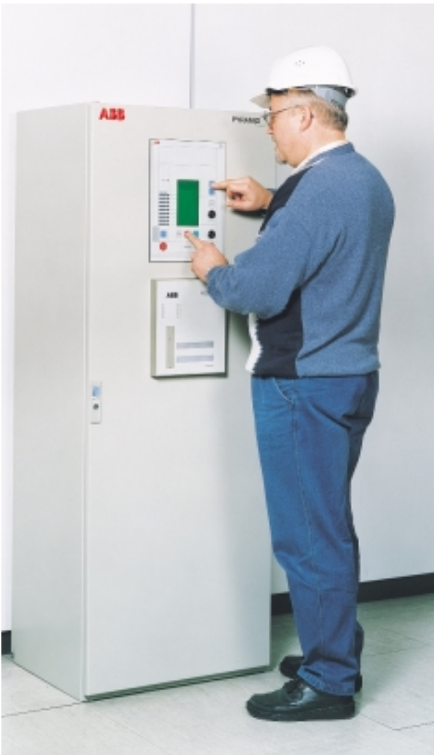
8 Compact control panel with SCU for a simple HV switchbay. Capabilities include back-up protection and additional main protection.
