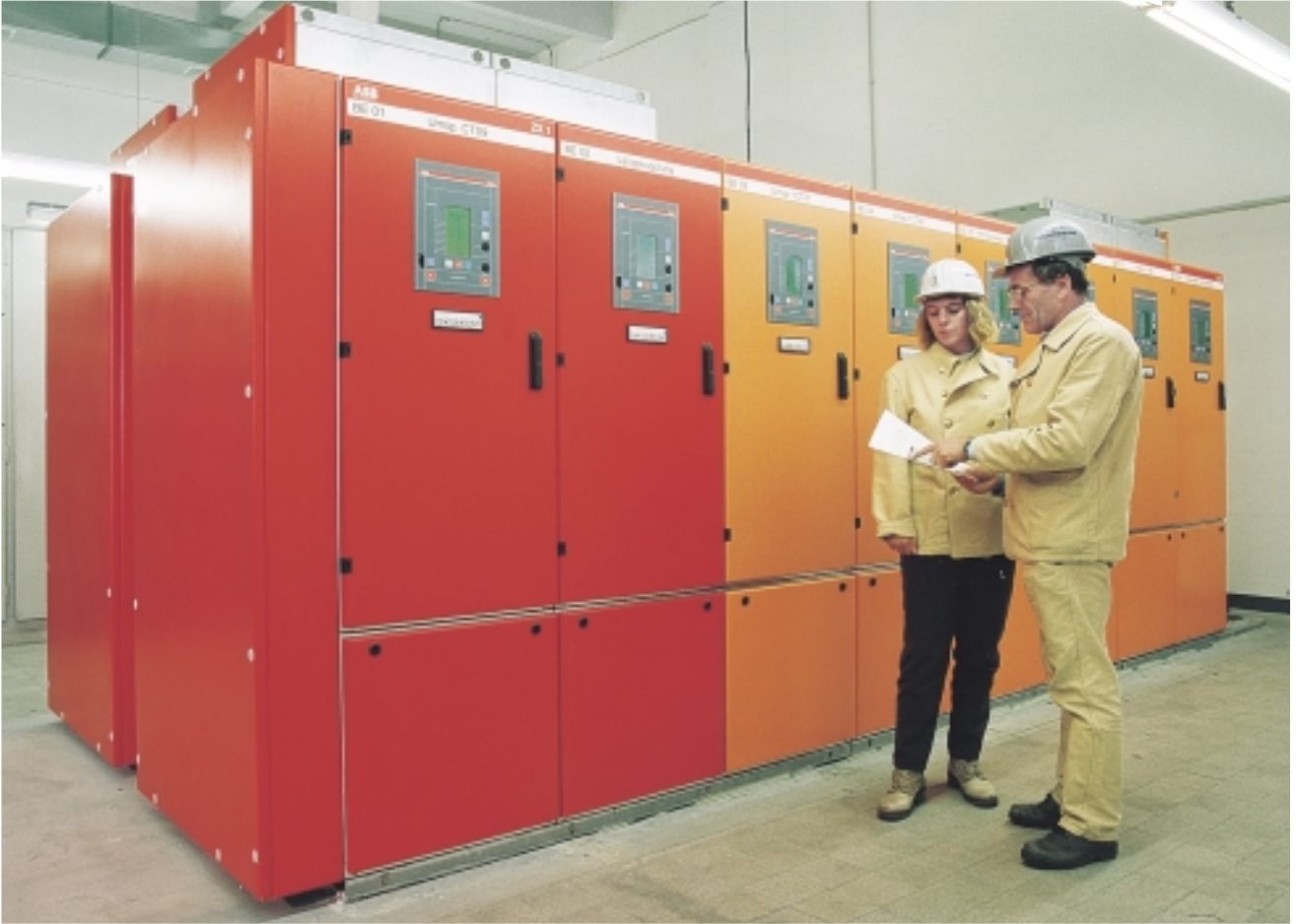
Medium-voltage substation with SCUs
