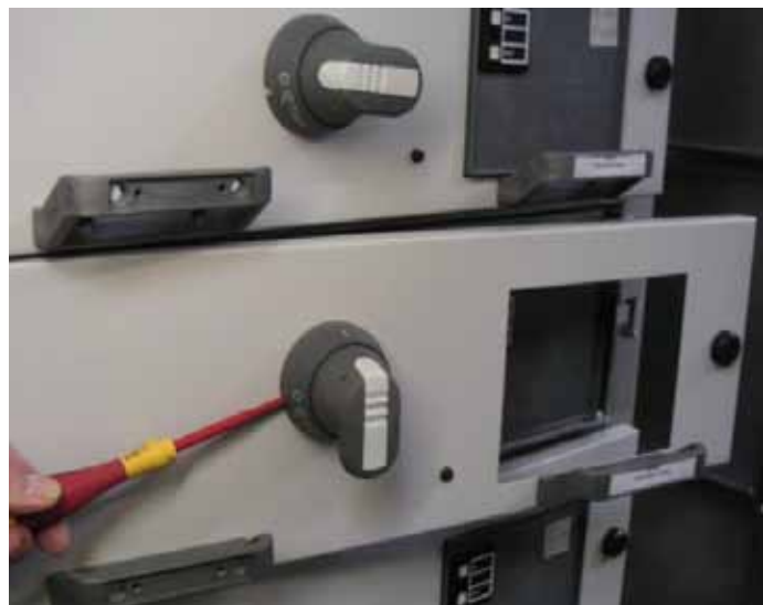
Fig. 45 Unlatching the front cover of a withdrawable module by means of a screw driver
