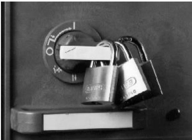
Fig. 40 Withdrawable module size 8E/4 with 3 padlocks
