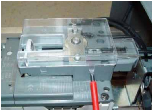
Fig. 1 and 2: Cover removal
