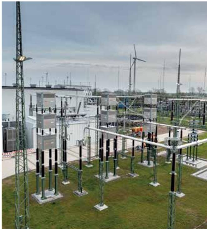
In any HVDC converter station, power losses are the main driver of environmental impact. Over the complete lifetime of a station, losses can account for more than 90 percent of the total climate change impact, depending on the country's energy mix. Civil and construction materials, constituting more than 80 percent of a converter station, have the second biggest impact.
