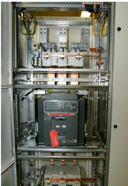
Incomer 3200A with air Emax circuit breaker and two earthing switches
