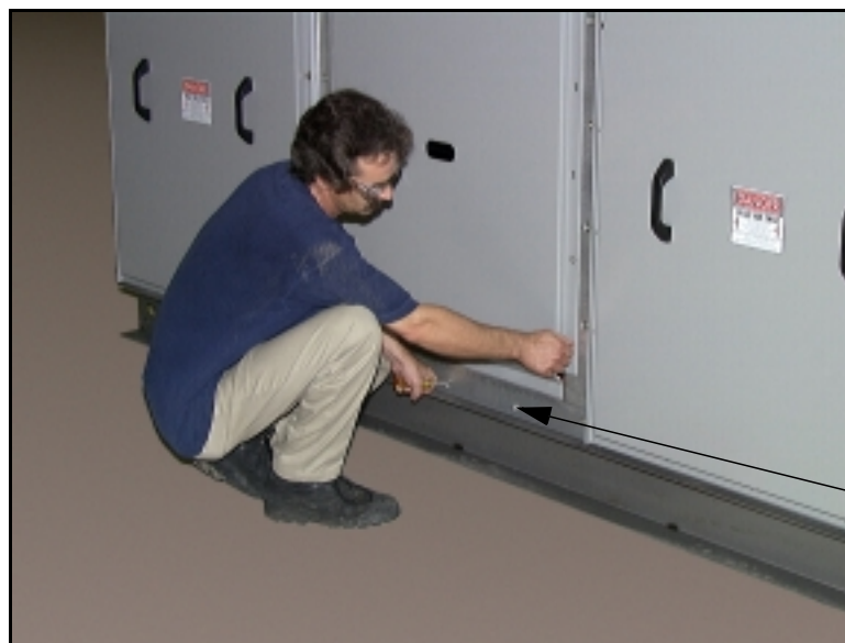
Figure 18: Step 4, Lower Inner Panel
