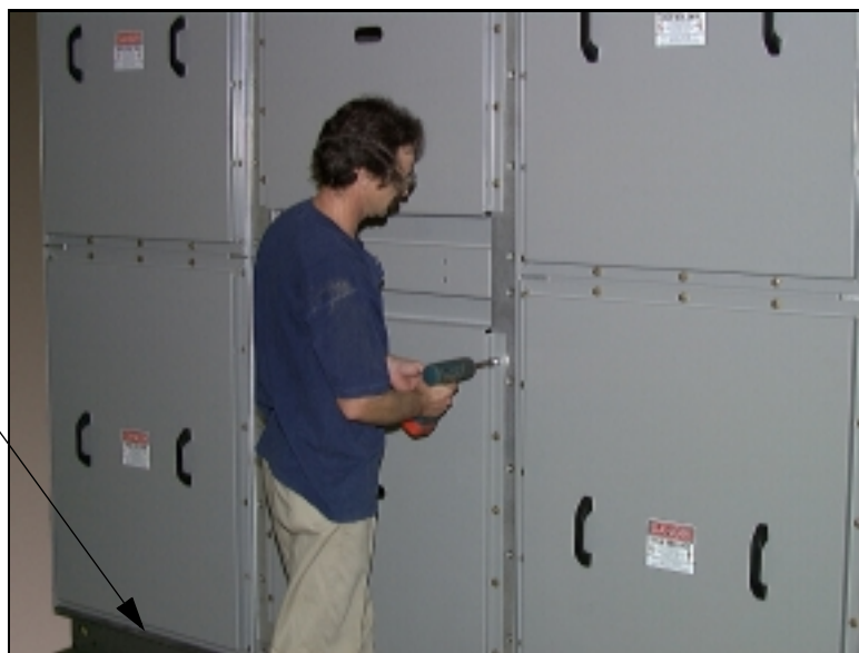
Figure 20: Step 5, Lower Inner Panel
