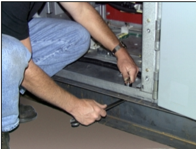
Figure 8: Unbolting the shipping base.
