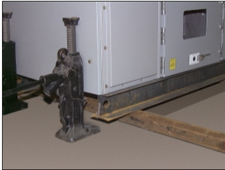
Figure 3: Position rollers under shipping base.
