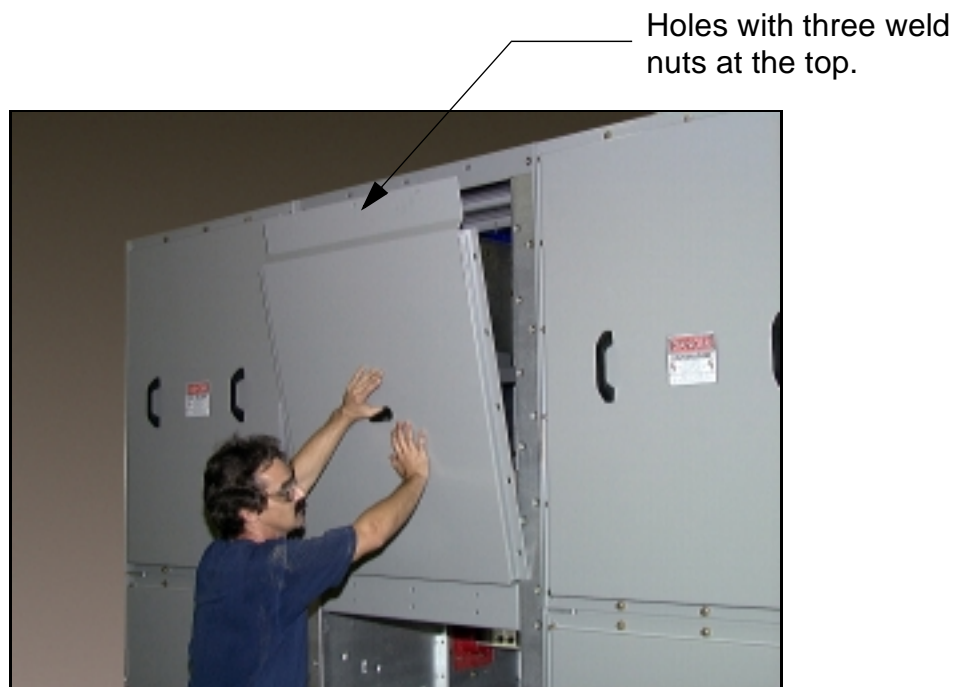
Figure 13: Step 1 and 2, Upper Inner Panel.
