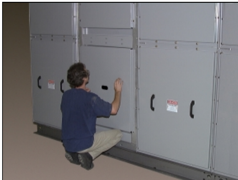
Figure 16: Step 3, Lower Inner Panel.
