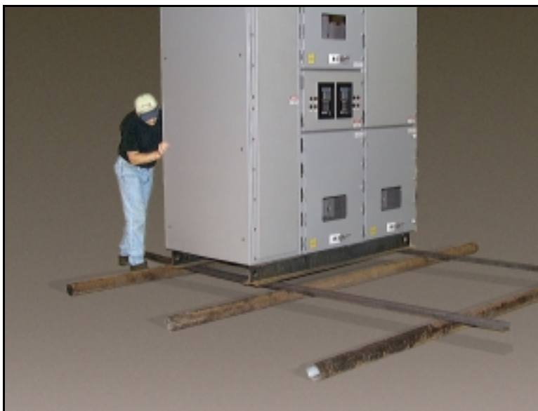
Figure 6: Carefully push the unit onto a third roller.
