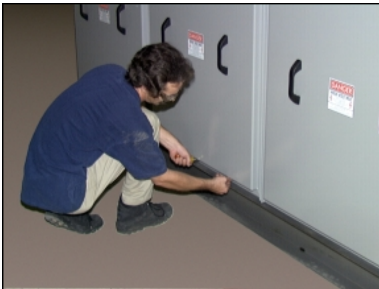
Figure 22: Step 6, Lower Exterior Panel
