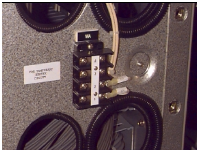
Figure 1: Heater load terminals. Remove before bolting sections together.
