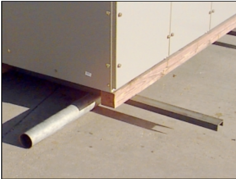
Figure 5: Position rails on rollers as shown for lateral moving.
