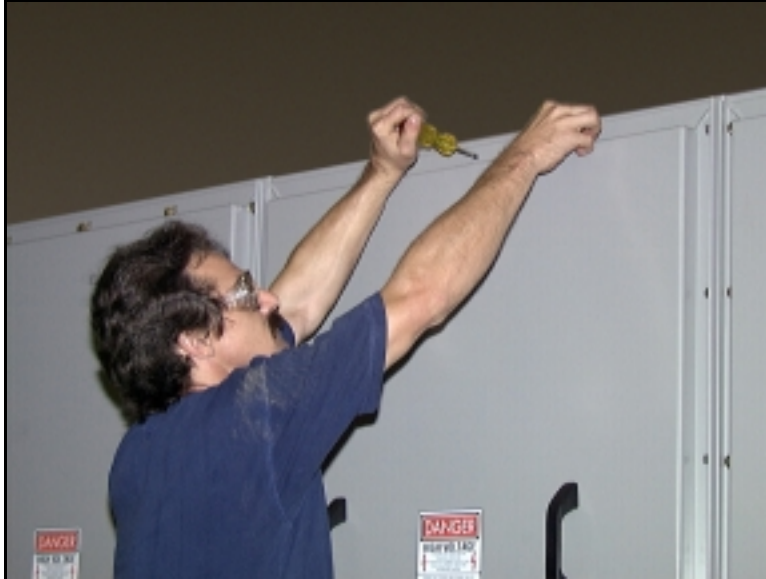
Figure 21: Step 6, Upper Exterior Panel
