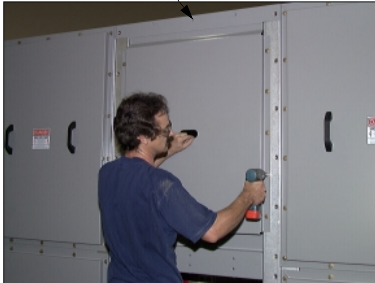
Figure 19: Step 5, Upper Inner Panel
