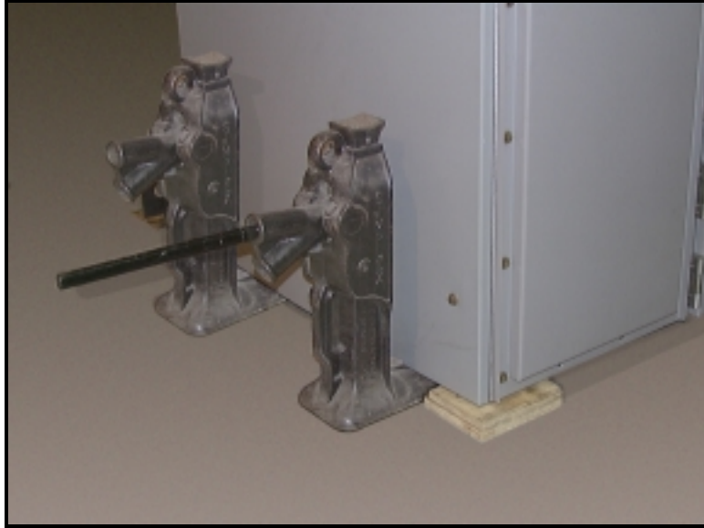
Figure 9: Lower the unit onto four pieces of wood.
