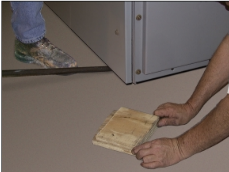
Figure 10: Use a pry-bar to remove the pieces of wood.
