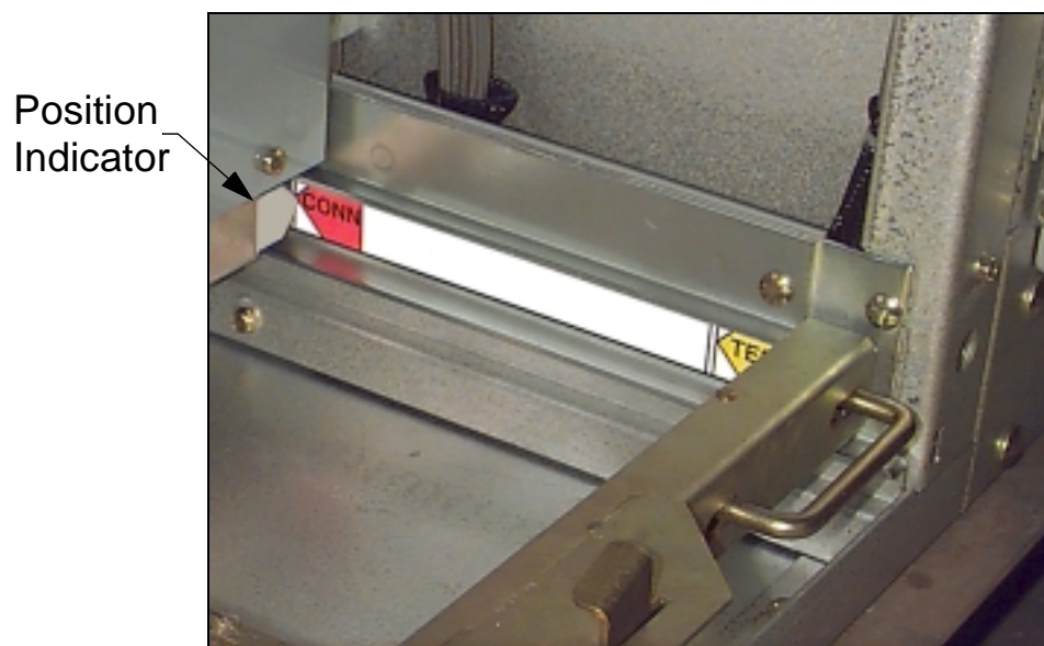
Figure 27: Circuit breaker position indicator.
