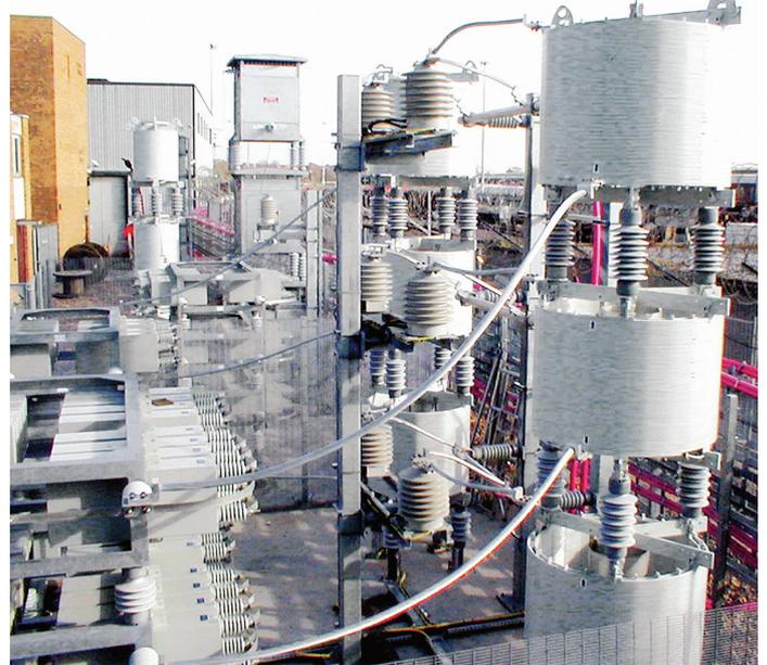
The 22kV transmission and 11kV distribution London Underground power supplies are converted by local transformer rectifiers to provide 630V/750V DC for the train motive power. The transformers also provide lower voltage supplies for lighting, lifts, escalators, ticket barriers, communications and control systems and so on.
