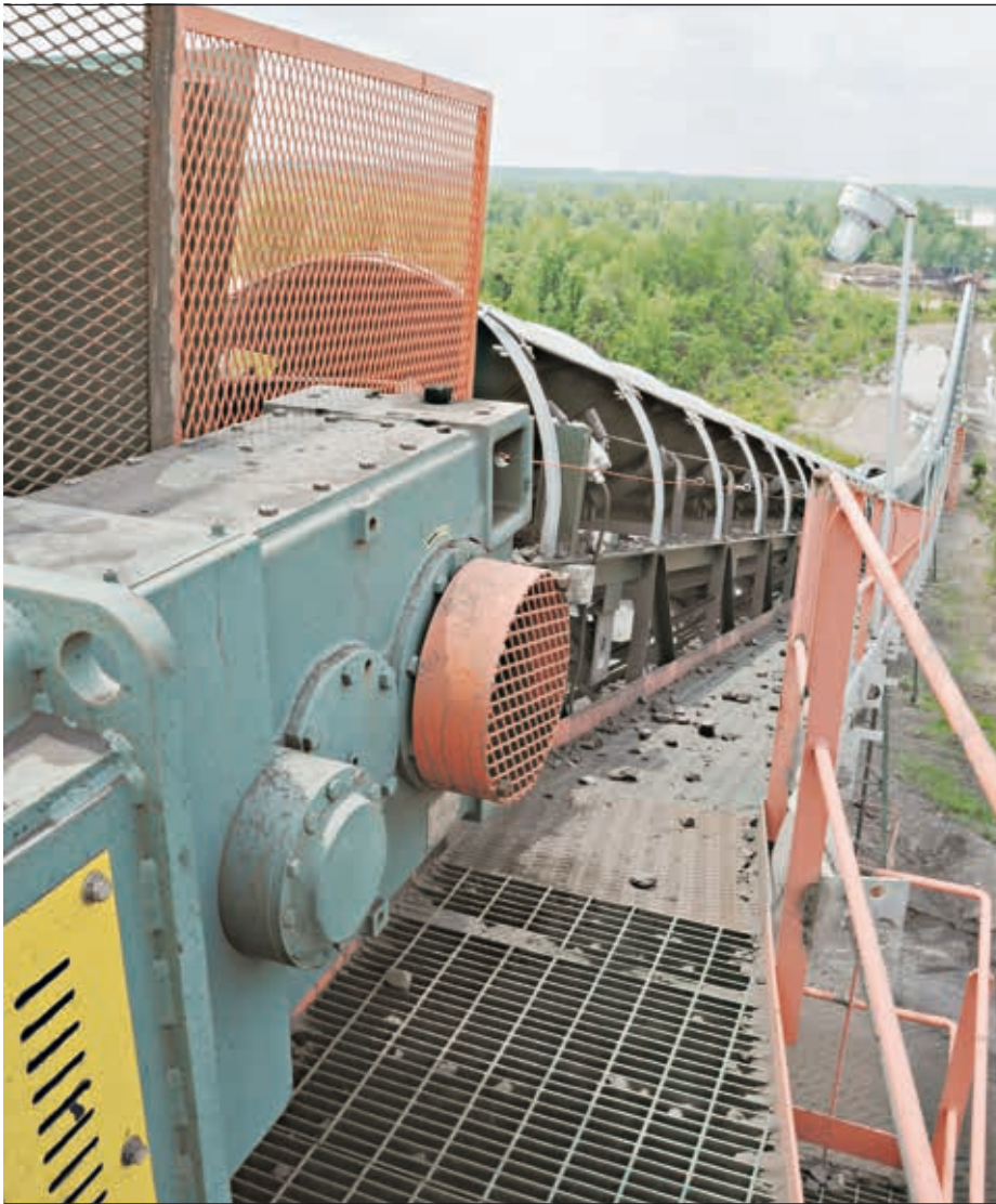
2 A 210K MagnaGear XTR operating on a 365 m long conveyor with a 26 m lift
