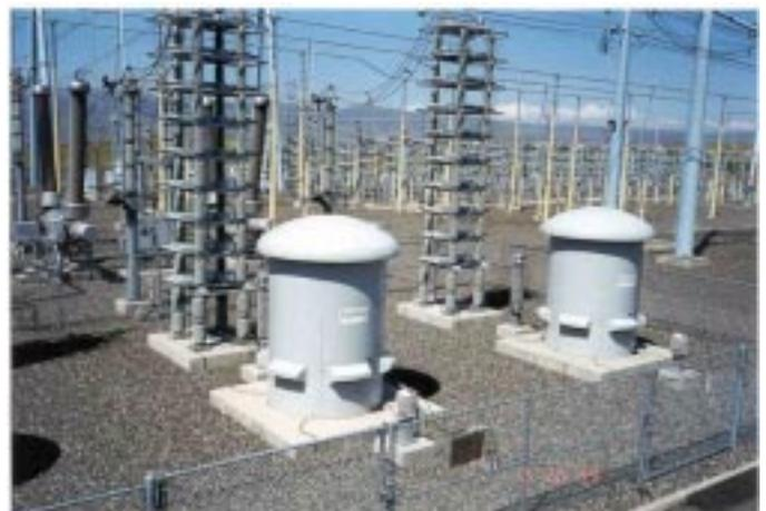
Fig. 4 ConTune filter installed in the Celilo station of the Pacific Intertie HVDC transmission, USA.
