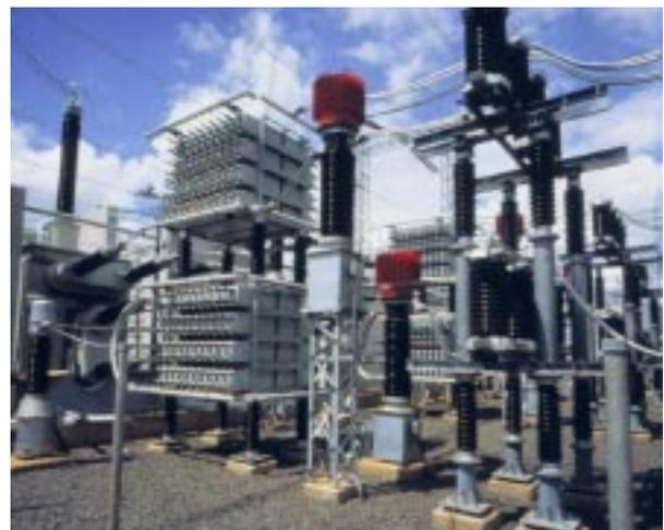
Fig. 7 Commutation capacitors at Garabi, Brazil
