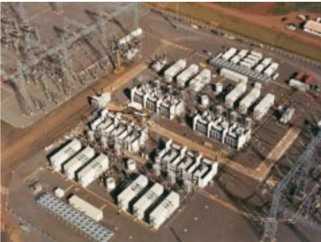
Fig. 8 Overview over the central part of two blocks in the Garabi 4\*550 MW back-to-back station, Brazil.
