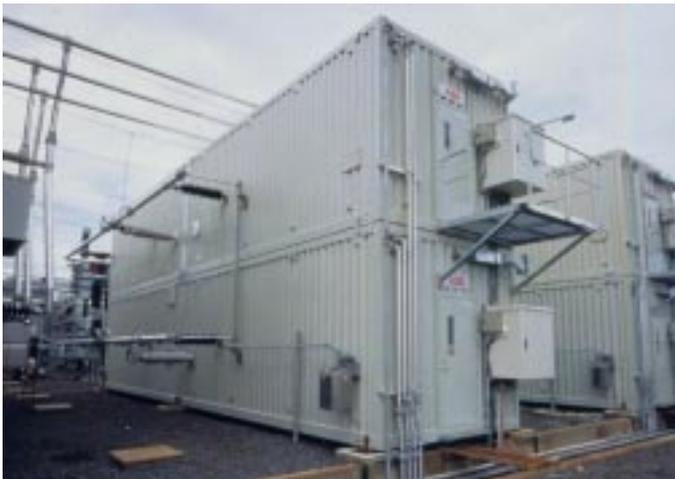
Fig. 2 The outdoor HVDC valves at Garabi are placed on top of each other to save space.
