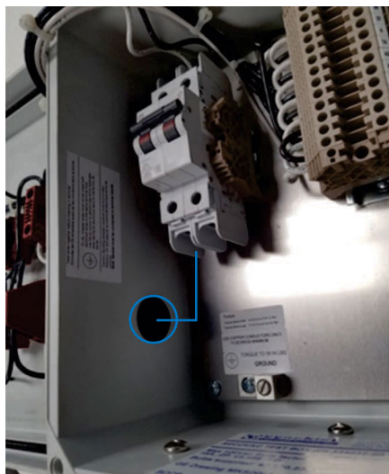
Figure 3-3: Incoming Power (Customer Provided)
