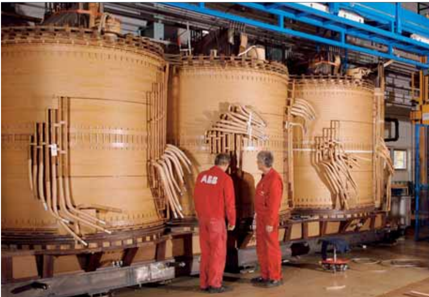
Repairing an HVDC transformer in Drommen, Norway
