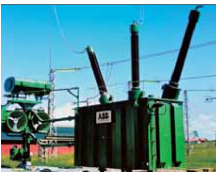
8 A 150 Mvar shunt reactor in the Swedish 400 kV grid
