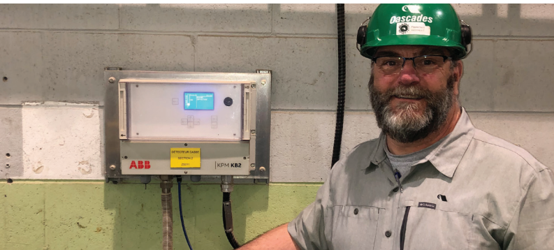
01 Mark Payeur by the KB2 electronics unit, which is always mounted outside the machine.
