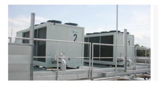
Rhoss, Italy. New motor starting solution from ABB reduced inrush currents of scroll compressors by 60 percent.
