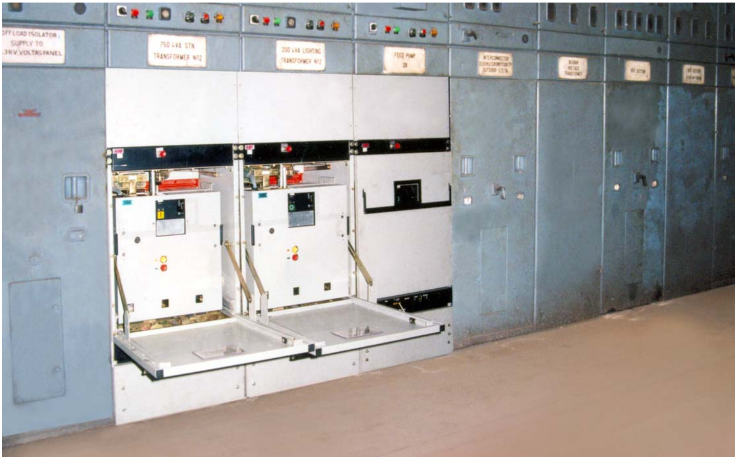
Retrofit of Reyrolle air blast circuit breakers with ABB SF6 circuit breakers
