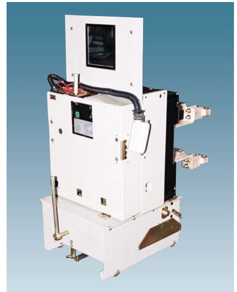
Voltas SF6 circuit breaker retrofitted with ABB SF6 circuit breaker
