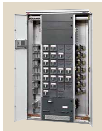
Motor control center
