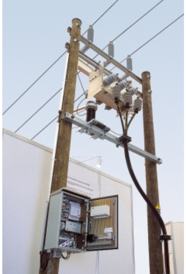
Pole-mounted, gas-insulated switch remotely controlled by DLC communication 6
