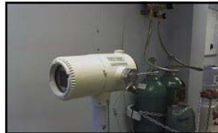
Installed NGC at South-Tex Treaters
