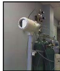
Installed NGC at South-Tex Treaters
