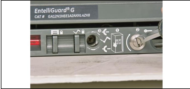
Figure 3.14. Racking Handle Shutter Drive Location
