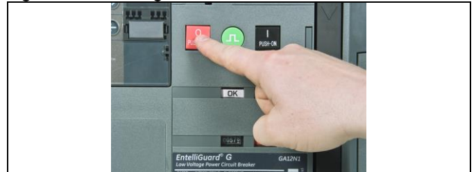
Figure 3.11. Setting the Circuit Breaker to OFF
