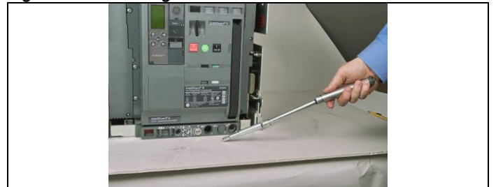
Figure 3.13. Racking Handle Extended
