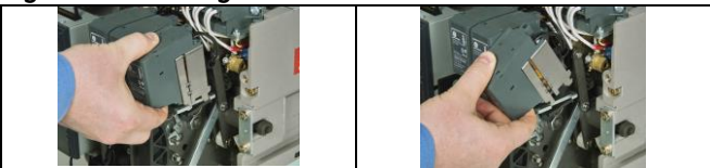
Figure 7.5. Closing Coil Installation
