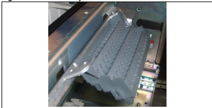
Figure 3.24. Secondary Disconnect
