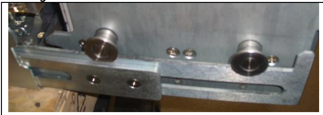
Figure 3.9. Circuit Breaker Rollers Straddled on the Loading Rails
