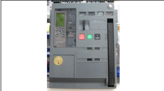
Figure 5.3. Key Lock for Breaker Trip Free Condition
