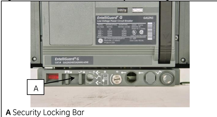
Figure 5.4. Circuit Breaker Security Padlocking Location
