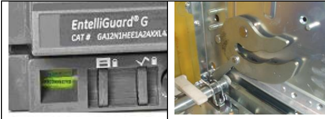
Figure 3.8. Racking Drive in the DISCONNECTED Position
