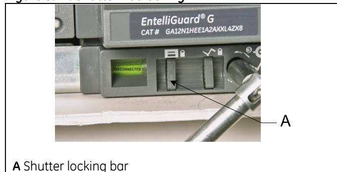
Figure 5.17. Shutter Padlocking
