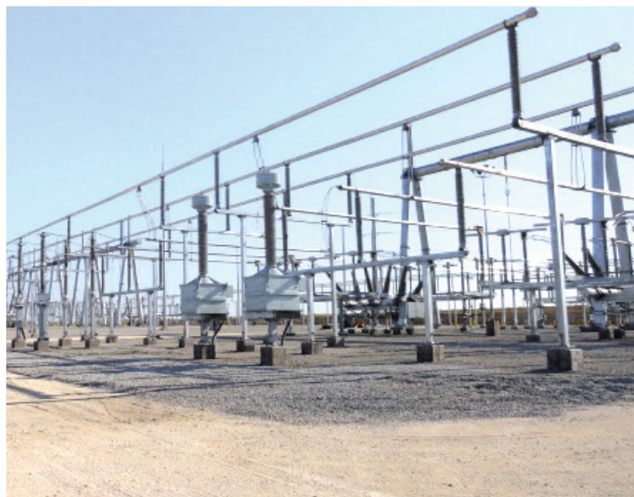
Products pictured left to right: STATCOM solution, manufactured in Switzerland, pictured at a wind farm in the United Kingdom, close-up: 345kV SSVTs in Texas.
