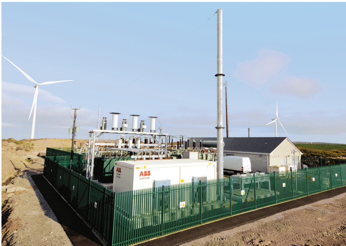
STATCOM solution, manufactured in New Berlin, Wisconsin, pictured at a windfarm in Puerto Rico.
