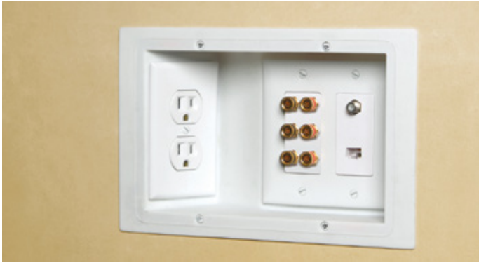
Ample room between drywall and studs
