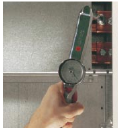
Connecting the horizontal busbars between the cubicle units with bolted joints is easy to carry out from the front.
