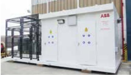
Switching operations are performed externally to provide the most compact design.
