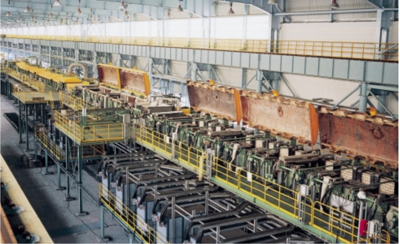
Pickling section of the annealing and pickling line at Baoyong Special Steel in Ningbo, China. The open tanks contain the rectifiers that generate the current flux used to clean the strip surface.
