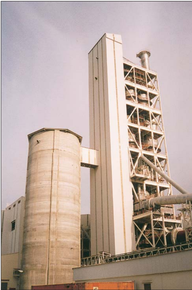
Raw meal blending silo and preheater tower.
