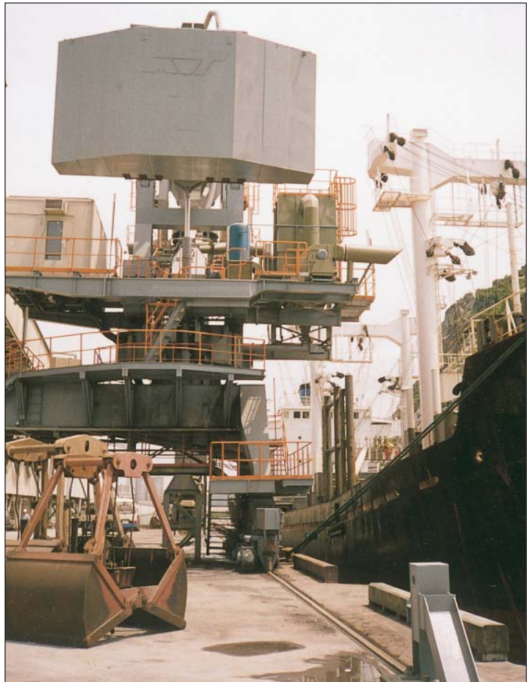
Ship unloader at the Hon Chong jetty.
