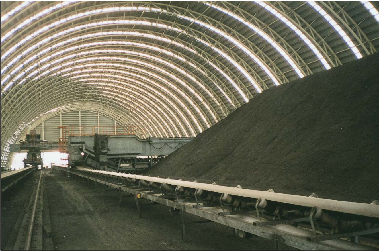
Coal storage building
