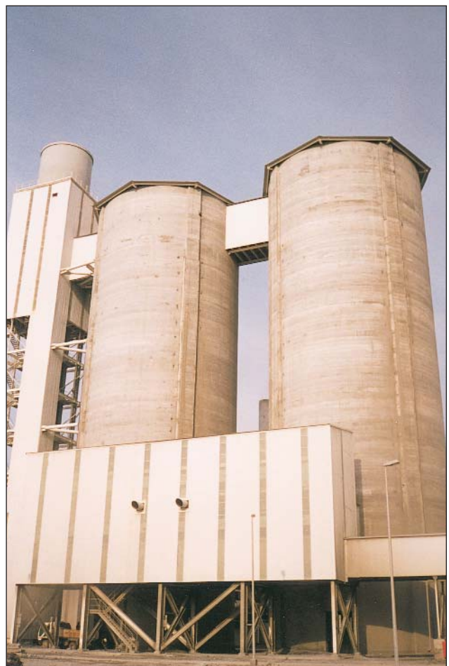
Cement storage silos.
