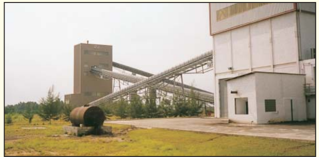
Pozzolana grinding plant building on the right with transfer tower in the background. Materials handling equipment and buildings were designed and built by FAM.
