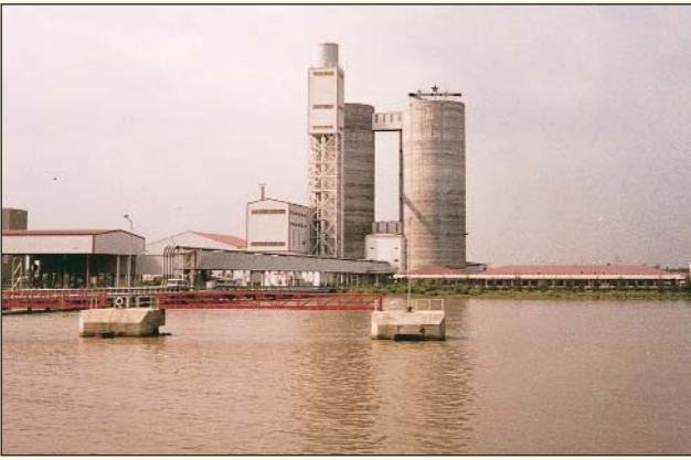
Approaching the terminal along the Dong Nai River. The 65 m high silos store ordinary Portland cement (right) and pozzolana blended cement (left).
