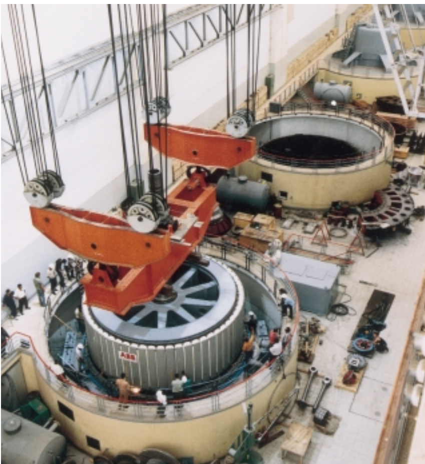
Lowering the rotor of generator no 4 into the stator
