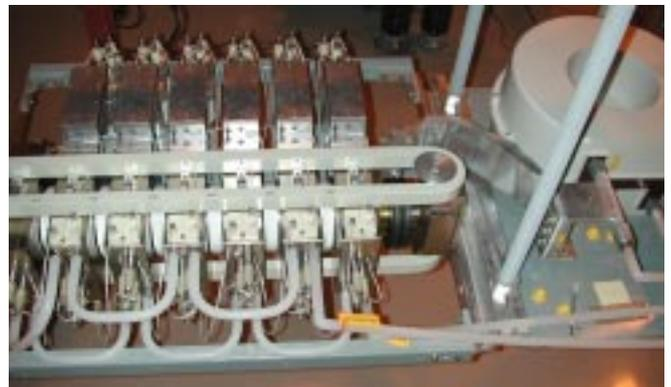
Fig. 1. One complete Garabi HVDC thyristor module
