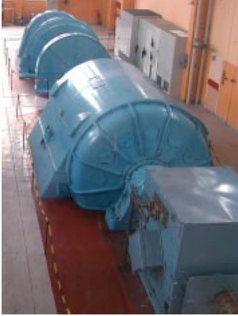
Fig.4 Test generator to feed the six-pulse Back-to-Back circuit
