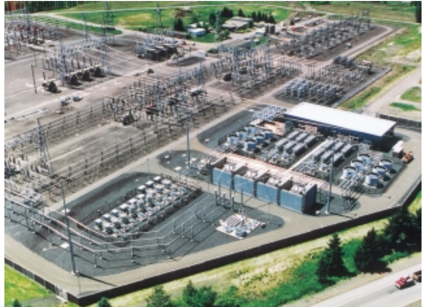
With the IGCTs, equipment designers can build more compact and less costly power control systems, eg static var compensators for utilities.
