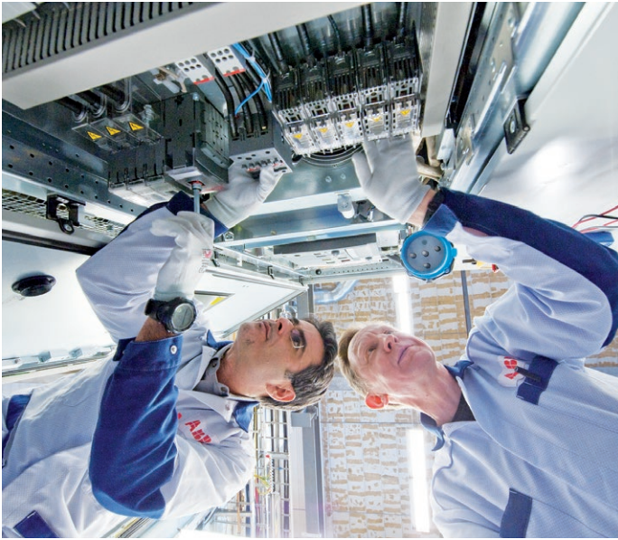
ABB engineers during workshop assembly
