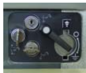
Interlocks on earthing switch operating mechanism
