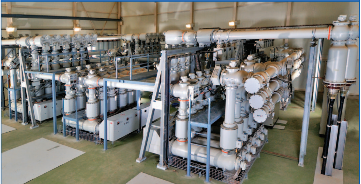
ABB's ELK-14, 300KV rated GIS
