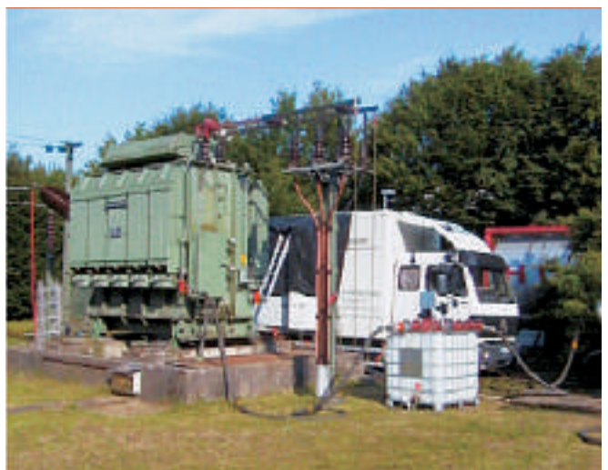
4 Mobile LFH unit for on-site transformer drying.
