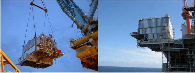
Figure 4. Lifting HVDC module and placed on platform.
