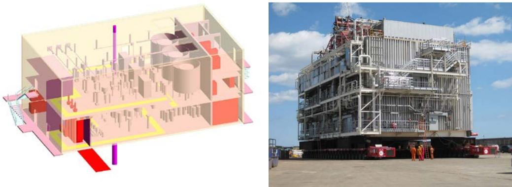
Figure 5: 3-D model of the Valhall offshore HVDC module and module at delivery from yard
