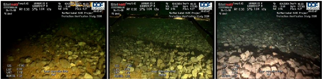
Figure 10 - Recently experienced trawl scars in dumped rock protection
