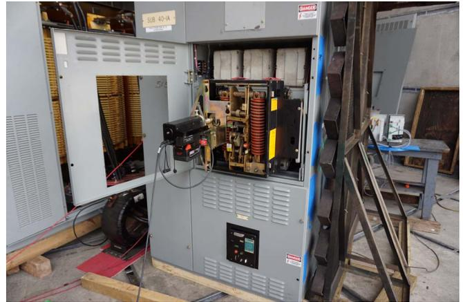
Fig. 16. Remote racking device used for line side fault of main circuit breaker.
