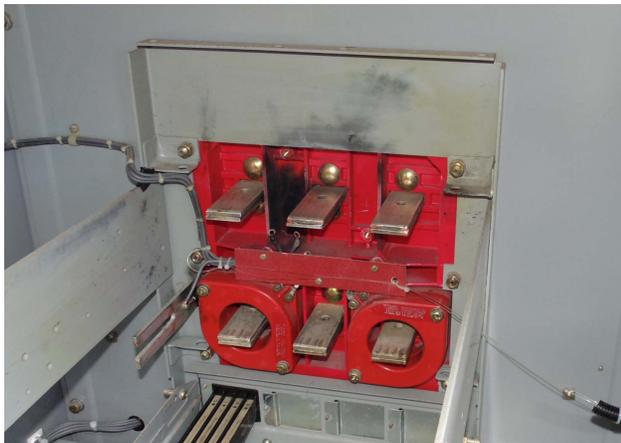
Fig. 15 Photo of damage to feeder compartment after arc fault with HSGS protection.
