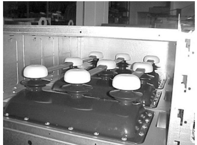
Figure 3.28 Aluminum field control caps covered by EPDM-rubber caps.
