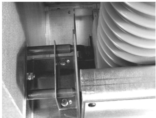
Figure 5.5 Sliding circuit-breaker to the leader.
