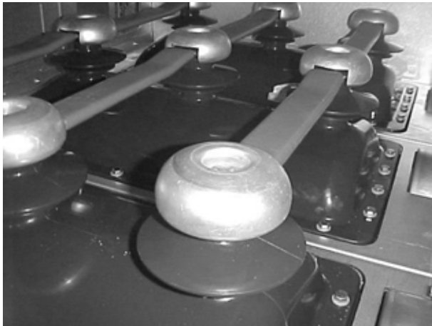
Figure 3.27 Aluminum field control caps.
