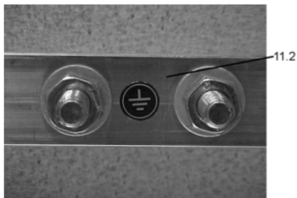
Figure 4.13 Position of earth symbol.
