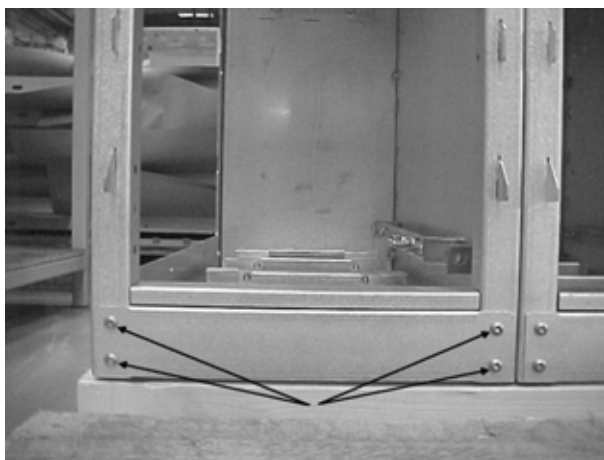
Figure 4.1 Screws on the base plate.
