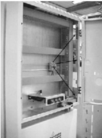
Figure 3.15 Holes in the secondary compartment.
