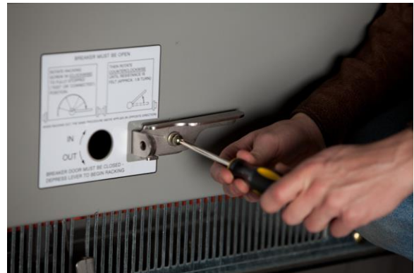
Figure 34: Removal of the Position Release Lever
