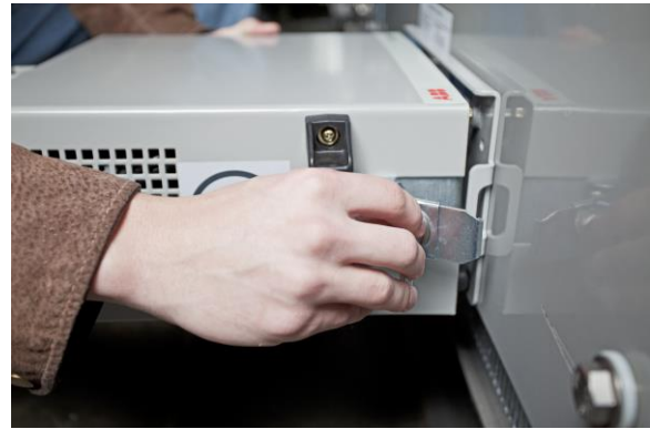
Figure 19a: Installation of Motor Box 1
