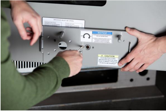
Figure 35: Installation of SmartRack™ mounting adapter plate
