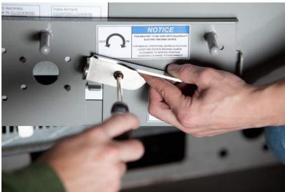
Figure 36: Installation of Position Release Lever
