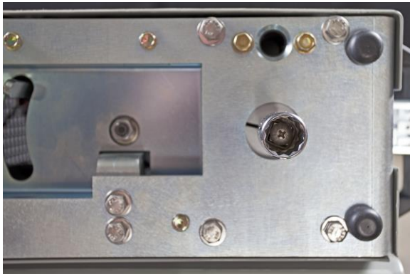
Figure 12: Racking Socket on Motor Box
