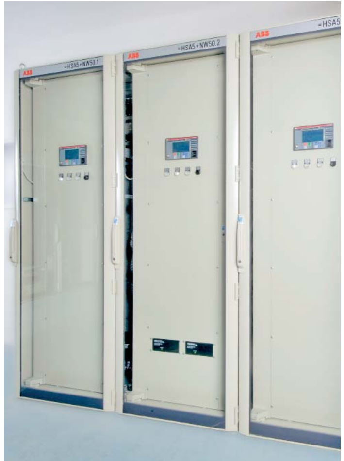
SUE ensures uninterrupted power supply at PCK Raffinerie GmbH – reliable and fault-free for generations.
